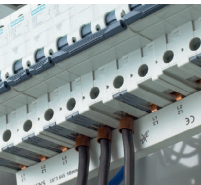
Clear connection of the feeder in front of the busbar.
